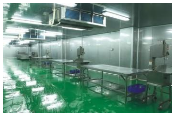
初加工区 Primary processing area
